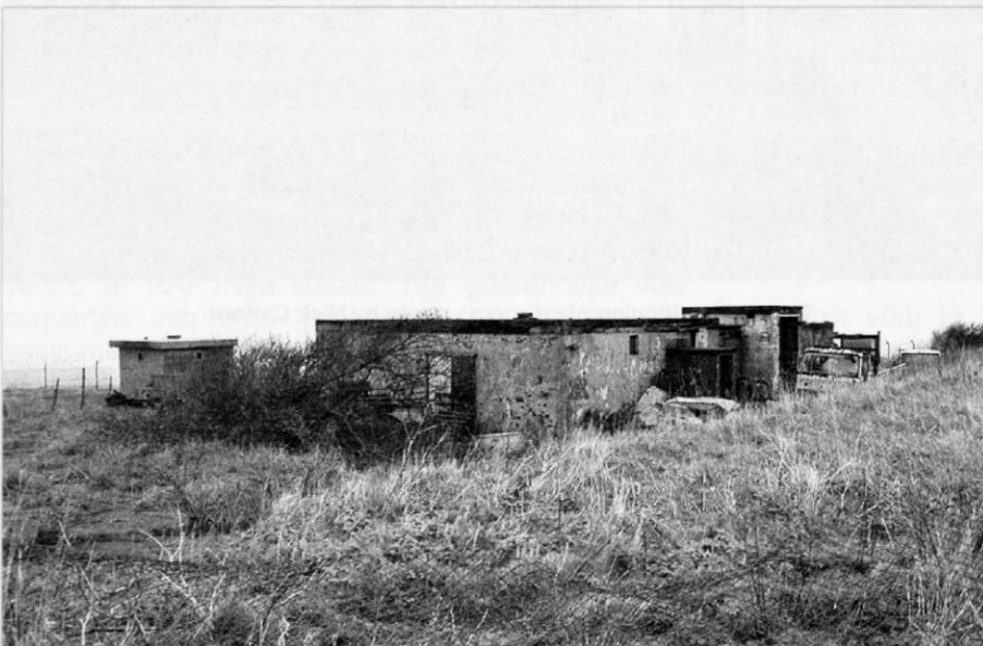
The Type 80 modulator building - Photo Dan McKenzie
